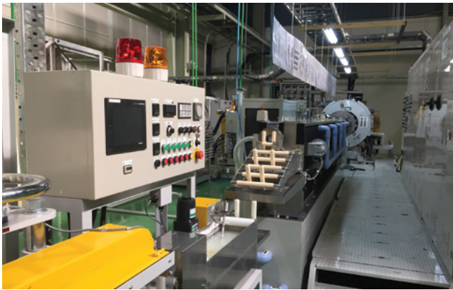
Commissioning of Alloy Wheel & Rubber Hoses Plants at Bawal Region
